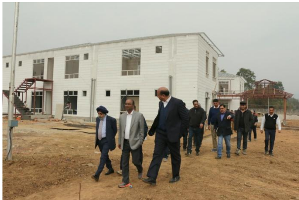
At Office complex and Residential complex, Tumlingtar
