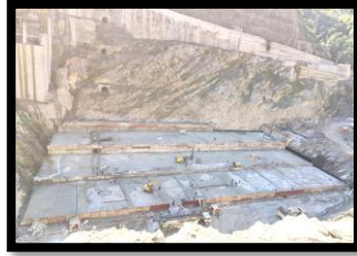
Dam Pit concreting
