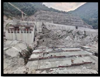
Left Bank Dam Stripping
