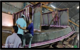
Radial Gate Inspection at Kota
