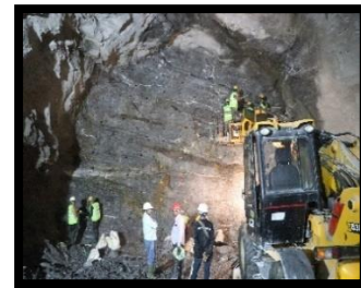
HRT Face-7 Heading
