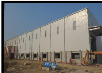
Substation work at Dhalkebar
