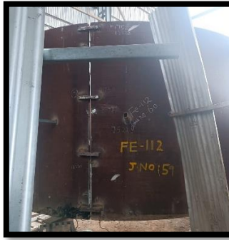
HM works at workshop
