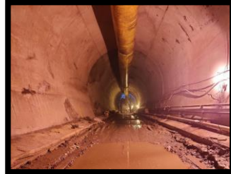
HRT Face 2 Overt Lining
