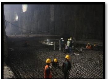
PH machine hall Reinforcement work in progress
