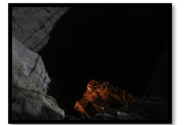
Gate Shaft 4 Breakthrough
