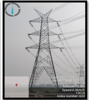
Tower Stringing Work
