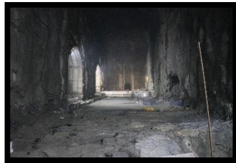
Transformer Hall Raft concrete work in progress
