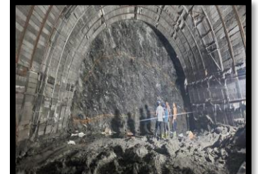
HRT Face-3 Heading
