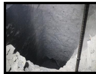
Gate Shaft 3 Breakthrough
