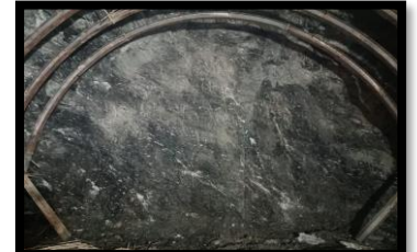
HRT Face-5 Heading
