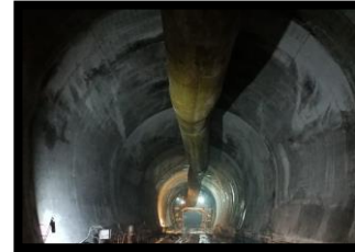
HRT Face-4 Overt Lining
