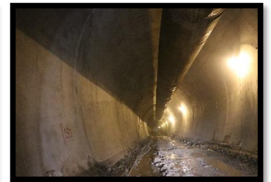
Face-7 Overt lining
