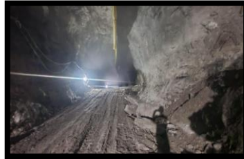
HRT Face-4 Benching
