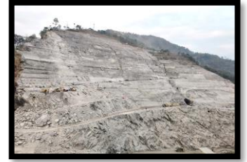
Right Bank Dam Stripping
