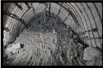
HRT Face-4 Heading
