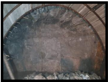
HRT Face-6 Heading
