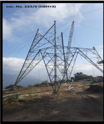
Tower Erection Work
