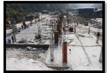
GIS Building 400 KV cable trench Raft concrete
