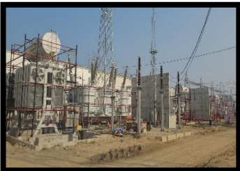
Substation work at Dhalkebar
