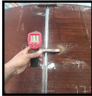
HM works at workshop
