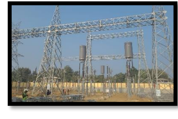
Substation work at Dhalkebar
