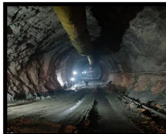
HRT Face-6 Benching
