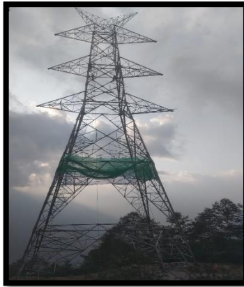
Tower Erection Work
