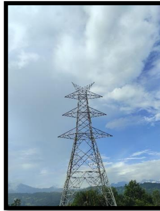
Tower Erection Work
