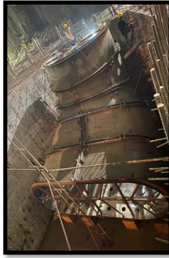
Unit#4 DT Cone welding in progress
