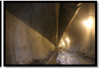
Face-7 Overt lining
