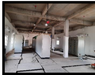
Substation work at Dhalkebar
