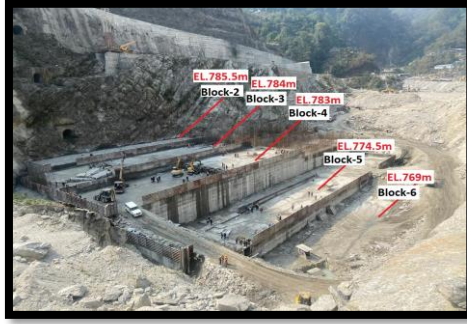
Dam Concreting
