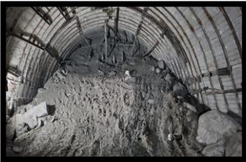
HRT Face-4 Heading
