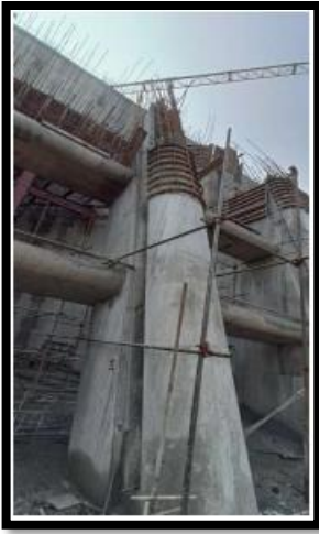
HM works Installation of Trash Rack Liner -Intake 1
