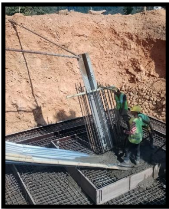
Tower Foundation Work
