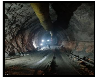
HRT Face-6 Benching
