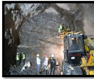
HRT Face-7 Heading
