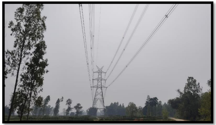
Tower Stringing Work
