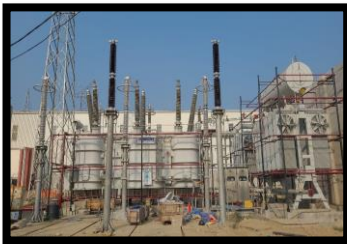
Substation work at Dhalkebar
