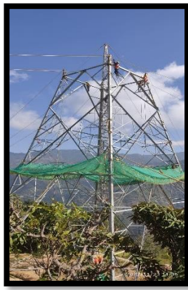
Tower Erection Work
