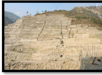
Right Bank Dam Stripping
