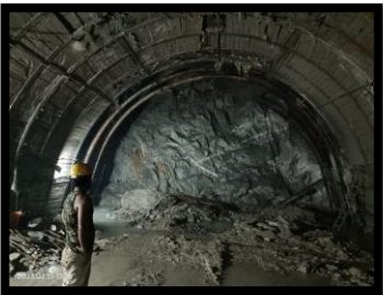
HRT Face-6 Heading
