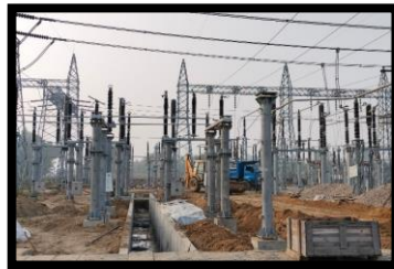
Substation work at Dhalkebar
