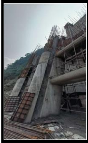
HM works Installation of Trash Rack Liner -Intake 2
