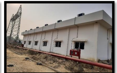
Substation work at Dhalkebar
