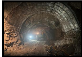
HRT Face-4 Benching
