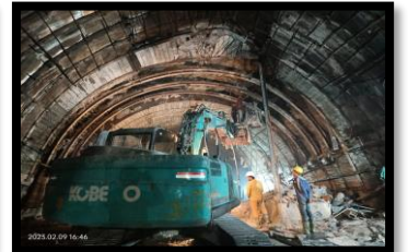
HRT Face-5 Heading
