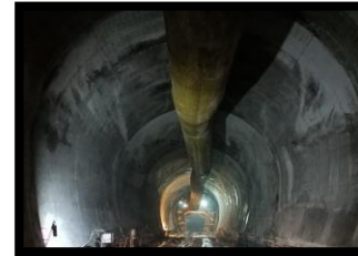
HRT Face-4 Overt Lining
