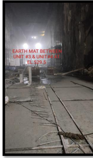
Earth Mat Laying between unit#3 & unit#4
