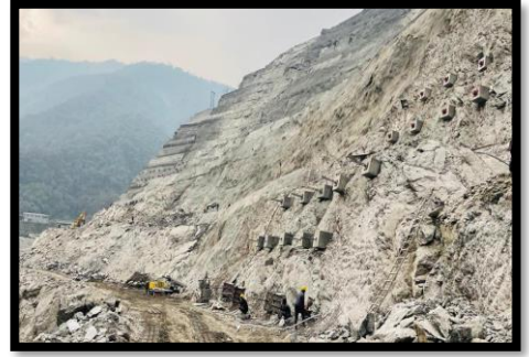
Dam Cable Anchors
