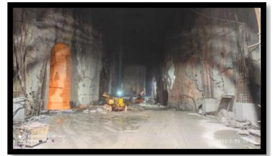
Transformer Hall Raft concrete work in progress
